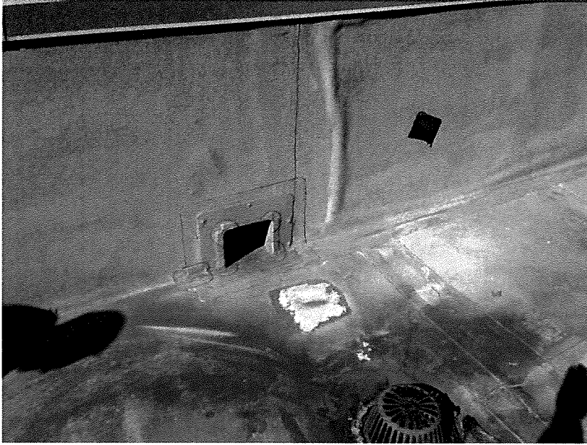
Internal roof drain with scupper overflow.
