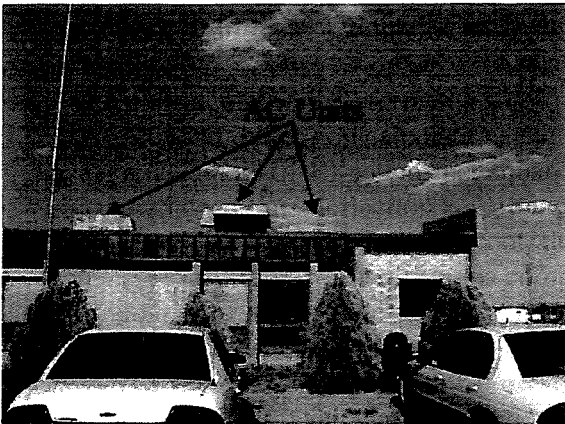
Photo #9: AC Units add to roof load
