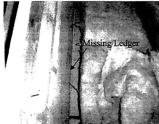
Photo #2: No ledger to support ceiling edge.
